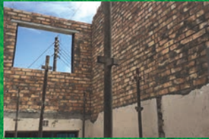
Safe House, Heideveld. The brick second storey is completed. (Nov16)
