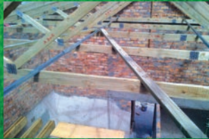
Safe House, Heideveld. The roof timbers in place. (Dec16)
