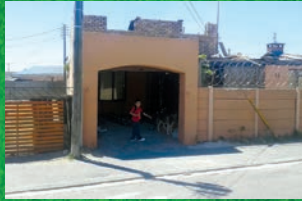
Safe House, Heideveld. Work begins. A home for six children. (Oct16)
